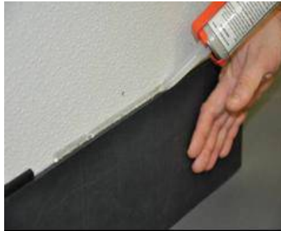
E6100 applied to top of base metal
