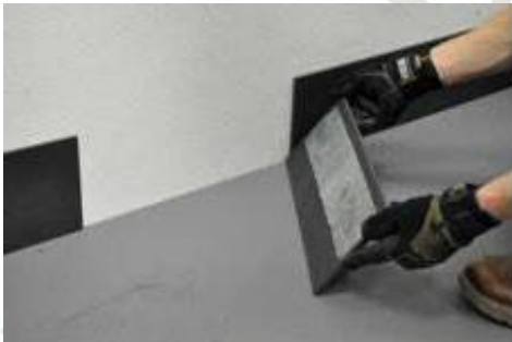
Using web reinforced tape
