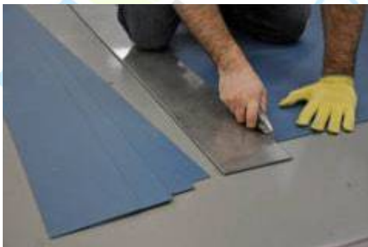
Turning 5' x 8' sheets into 6" x 8' strips
