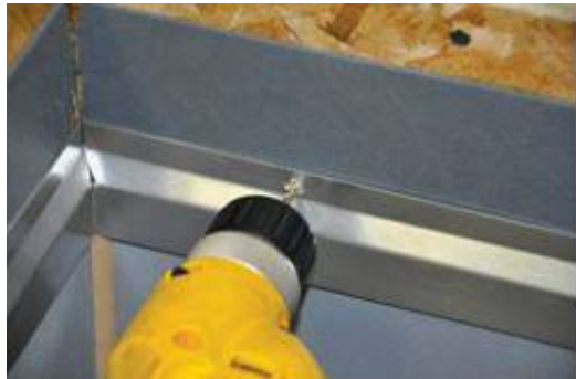
Pre-drill using 1/8" drill bit
