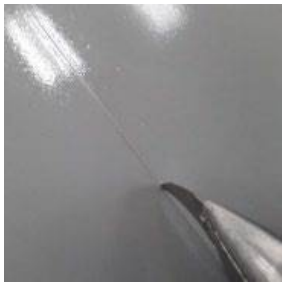
Cut through the applied tape
