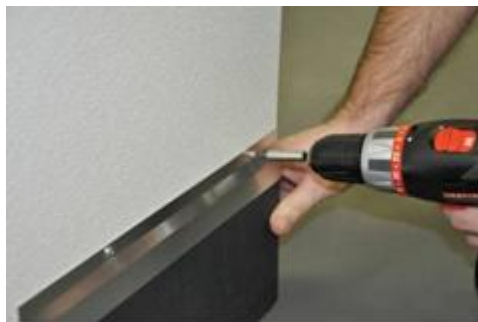
Image 21: Dry-fit Z-bar to wall.
