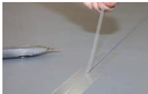
Image 3: Remove perforation
